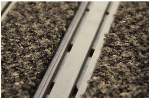
Entrance mats need to be rolled up periodically to allow the matwell to be thoroughly vacuumed. All stones and grit particles should be picked up.
