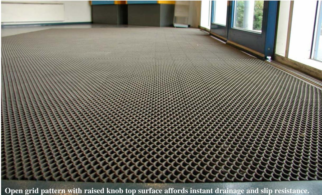
Open grid pattern with raised knob top surface affords instant drainage and slip resistance.
