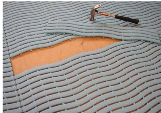
Ultima tiles can be connected easily with a hammer.
